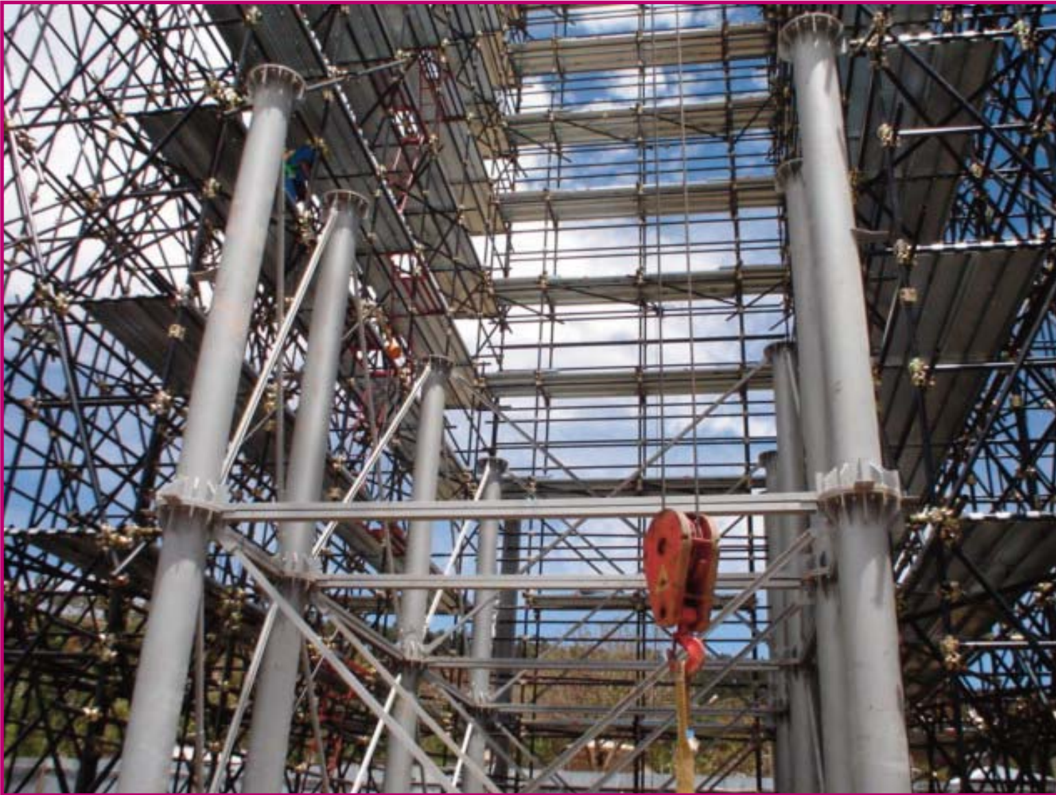
FIGURE 41 – THE STEEL TOWER, UNDER CONSTRUCTION, ON THE TOP OF WHICH THE BRIDGE CRAINE WILL BE HOUSED
