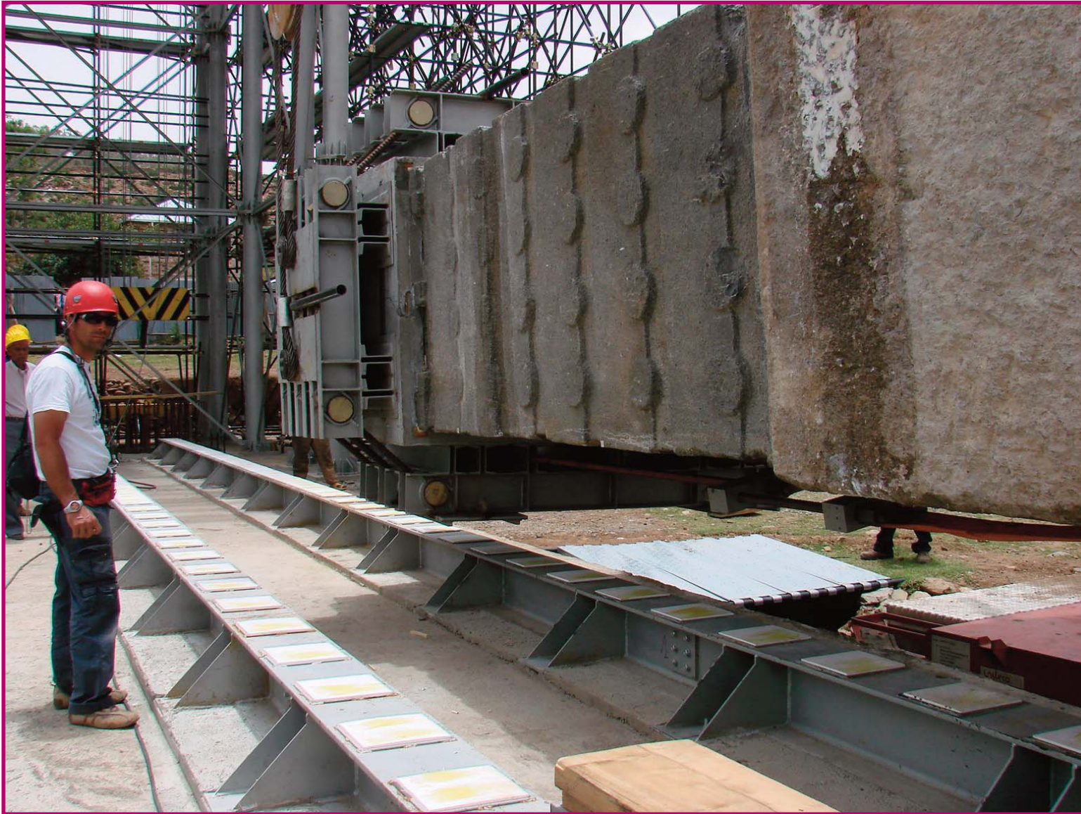
FIGURE 53 – THE BLOCK IS LOCATED ON THE RAILS.
