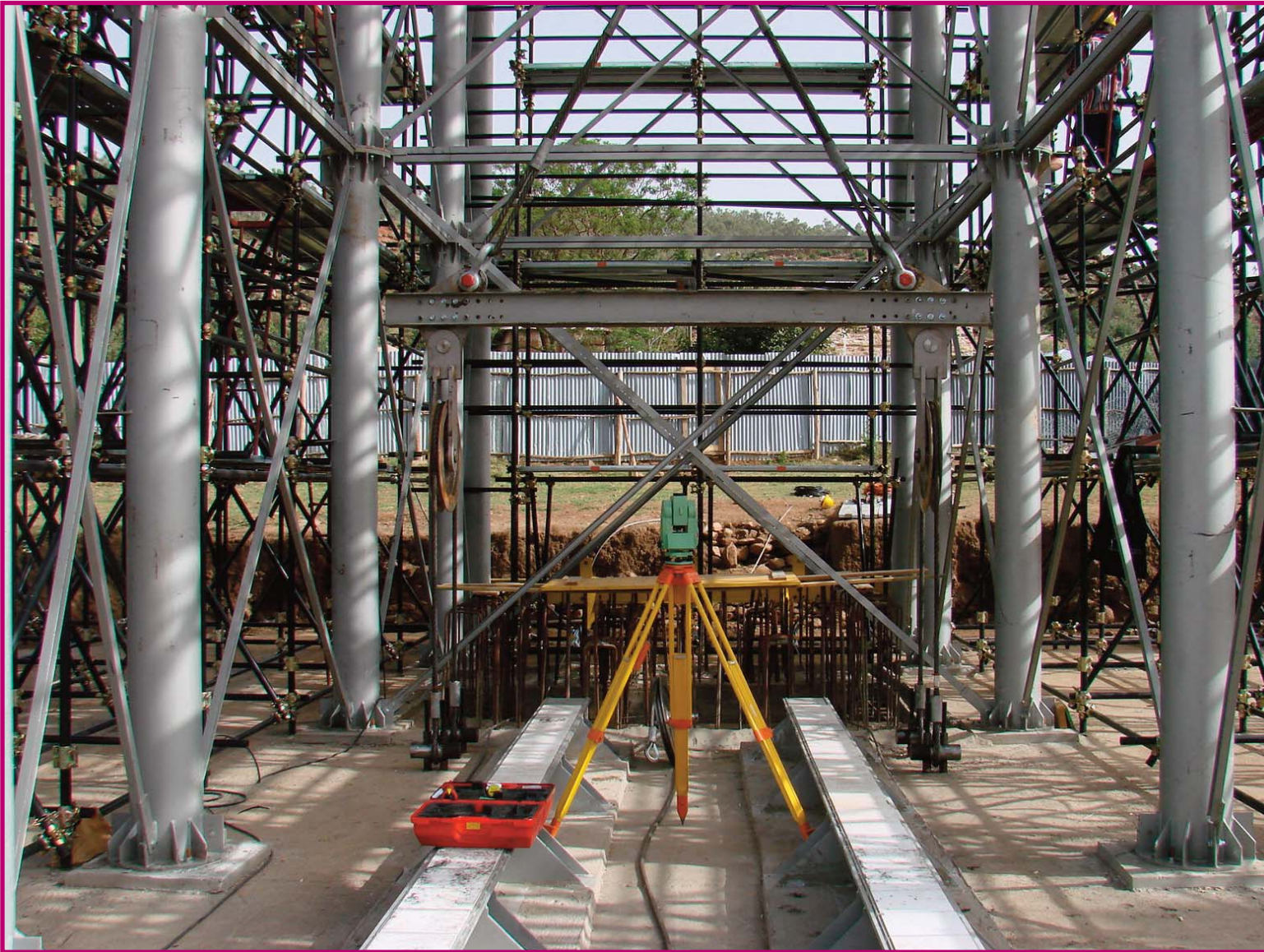
FIGURE 55 – PRECISION TOPOGRAPHIC SURVEY ENSURING VERTICALITY OF THE BLOCK.
