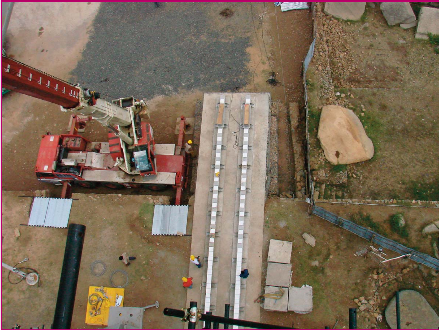
FIGURE 48 - THE RAILS USED TO SLIDE THE BLOCKS OF THE STELE.
