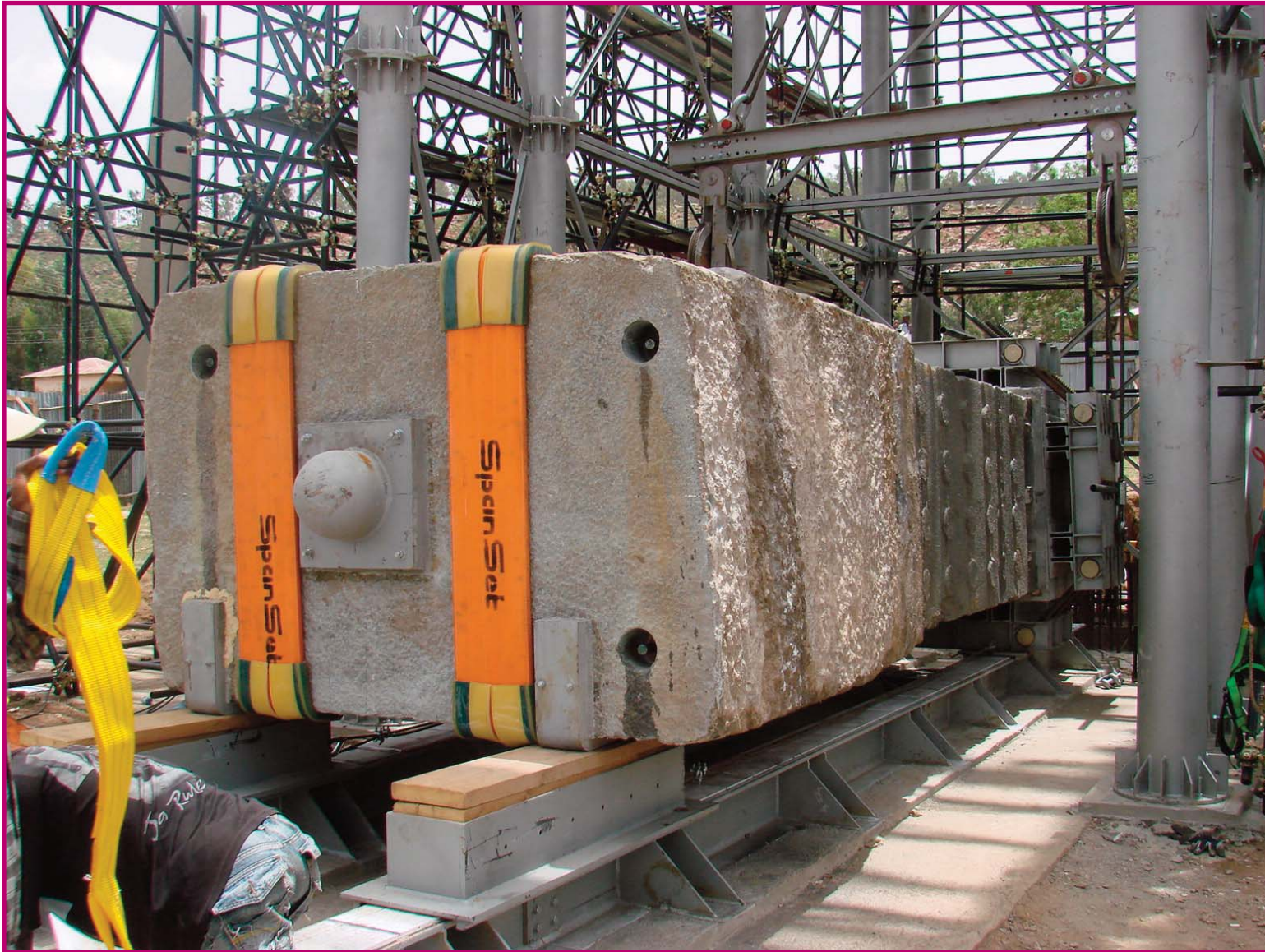
FIGURE 57 – THE BLOCK TO BE LOCATED IS MOVED INTO THE CASTLE.
