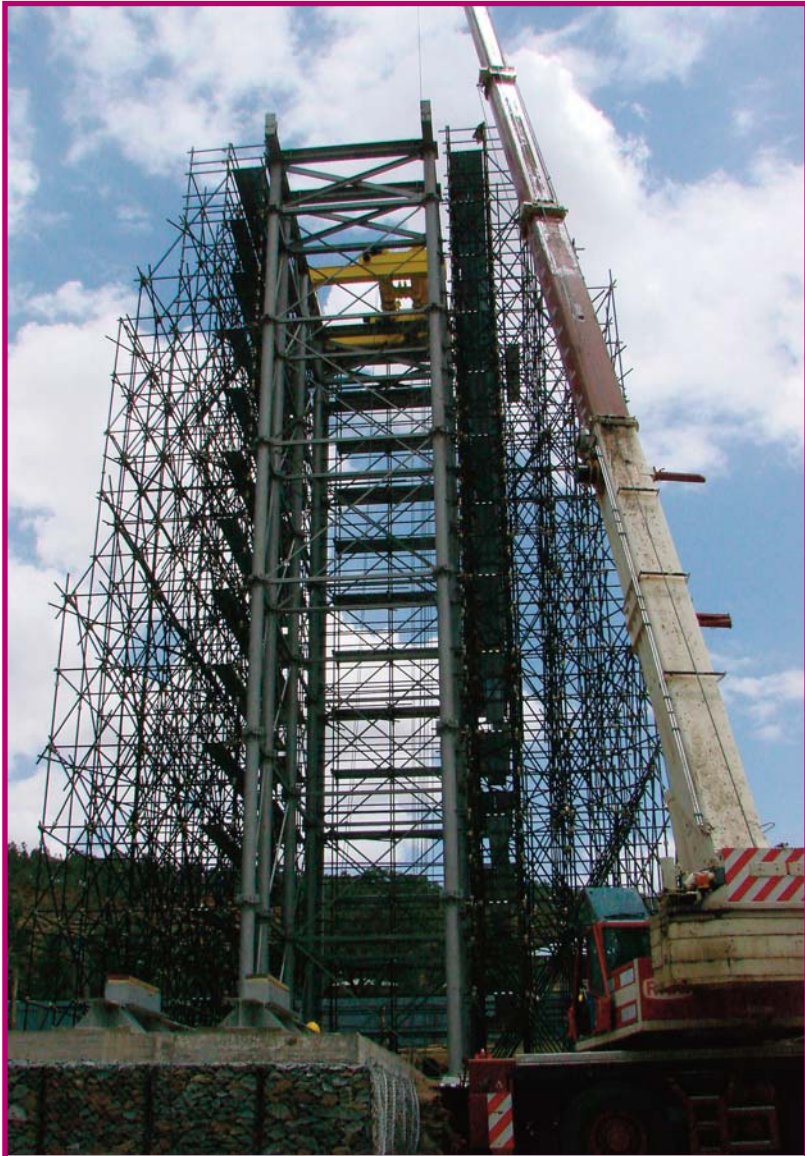
FIGURE 42 – THE STEEL CASTLE SUPPORTING THE BRIDGE CRAINE. FIGURE 43 – A JOINT OF THE STEEL CASTLE.
