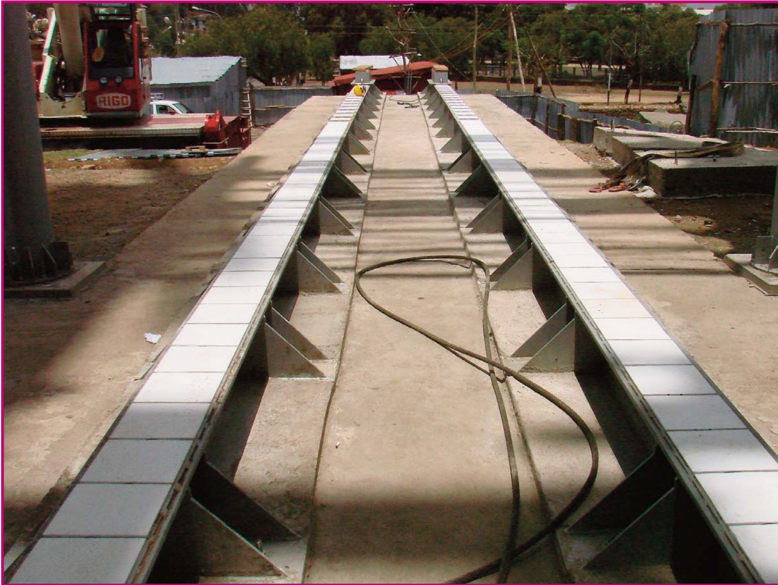
FIGURE 49 – THE RAILS USED TO SLIDE THE BLOCKS OF THE STELE: LOOK-UP.
