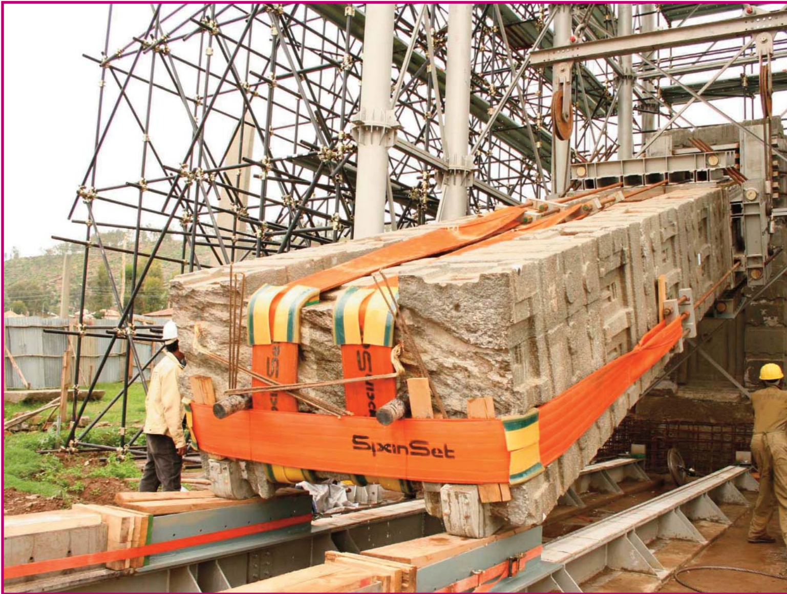
FIGURE 67 - THE SECOND BLOCK SLIDES ON THE PLATFORM FIGURE 68 - LIFTING UP OF THE SECOND BLOCK
