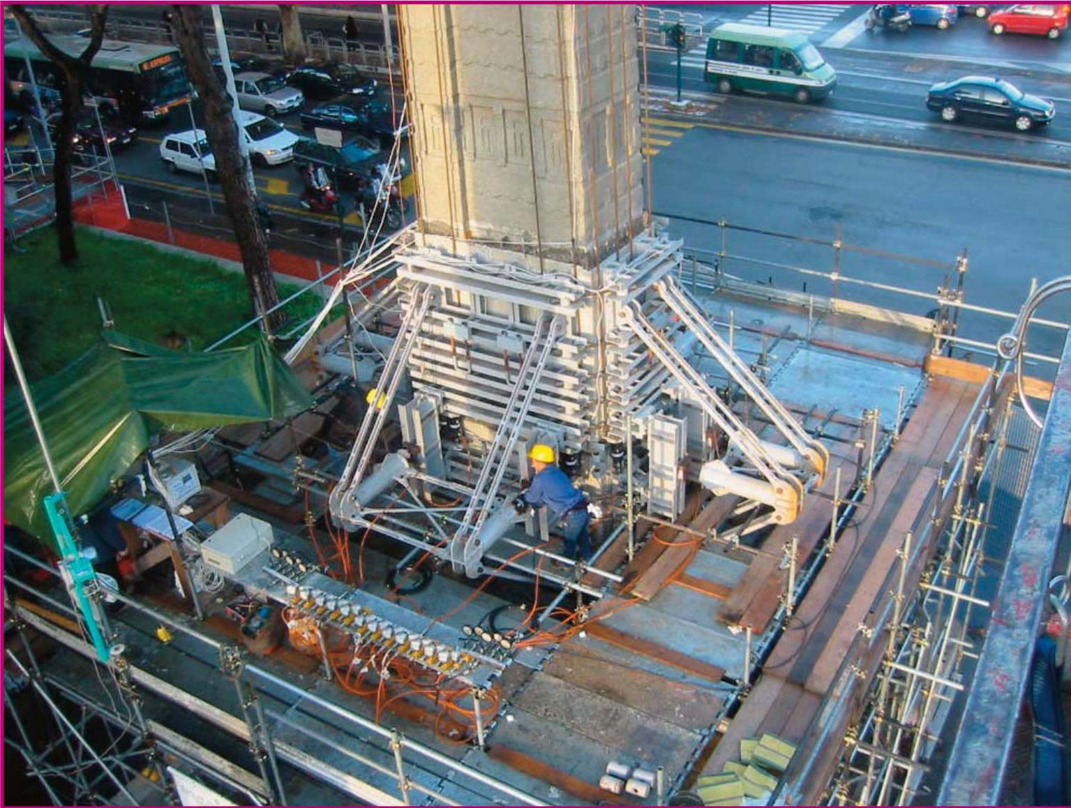
FIGURE 13 – THE STEEL STRUCTURE INCLUDING THE BRACES WHICH SUPPORT THE HORIZONTAL JACKS
