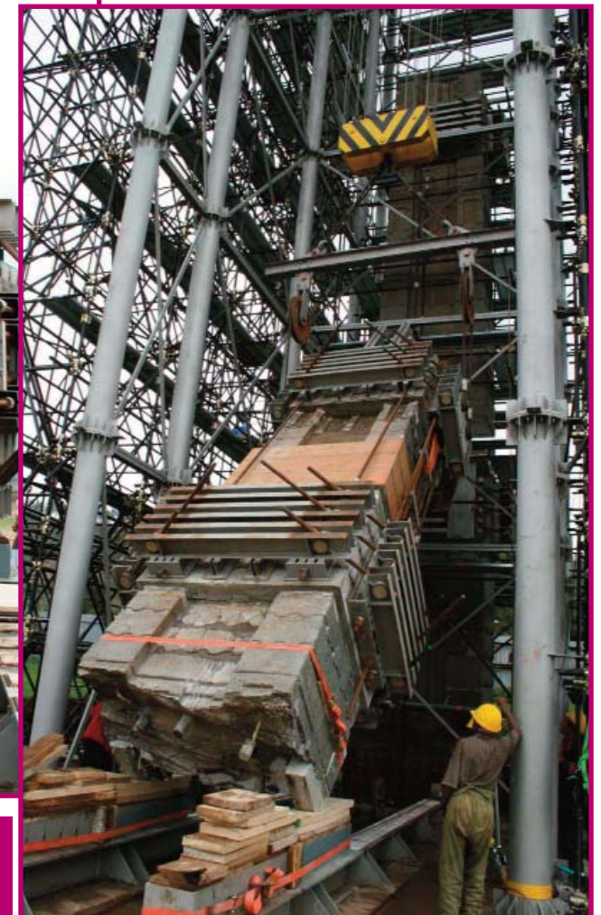
FIGURE 71 – THE LOWER PART OF THE THIRD BLOCK SLIDES ON THE PLATFORM WHILE THE UPPER PART IS LIFTED UP BY THE CRANE.
