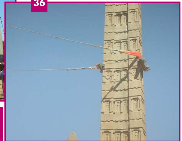
FIGURES 35, 36 – THE LEANING STELE N.3 AND THE INSTALLED REINFORCEMENT STRUCTURE MADE OF TWO INCLINED RAFTS AND CABLES FIGURE 37 – THE FOUNDATION OF THE RAFTS
