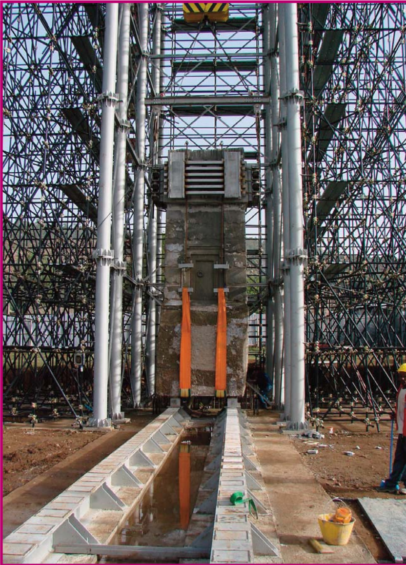
FIGURE 64 – LIFTING-UP OF THE BLOCK: LOOK-UP. FIGURE 65 – THE BLOCK IS MOVED TO THE FINAL VERTICAL POSITION AXIS.
