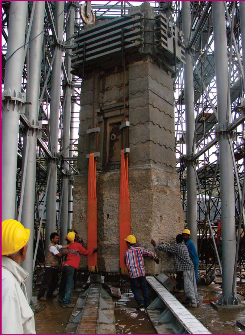
FIGURE 62 – THE BLOCK IS ROTATED AROUND ITS OWN AXIS. FIGURE 63 – LIFTING-UP OF THE BLOCK: GENERAL VIEW.
