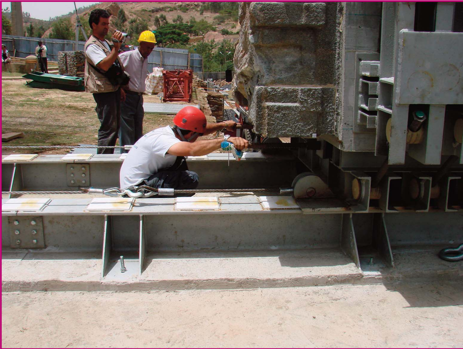
FIGURE 54 – FINAL POSITIONING OF THE BLOCK ON THE RAILS.
