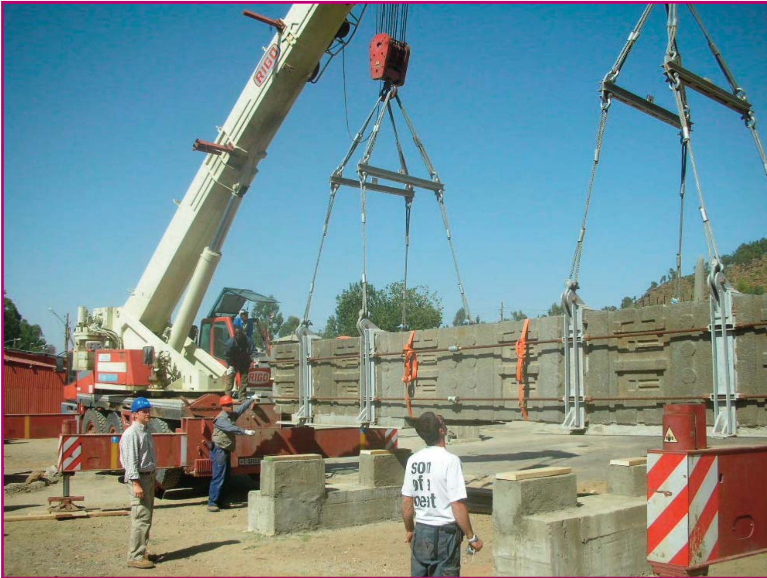
FIGURES 40 – HANDLING OF THE BLOCKS READY TO BE LIFTED UP
