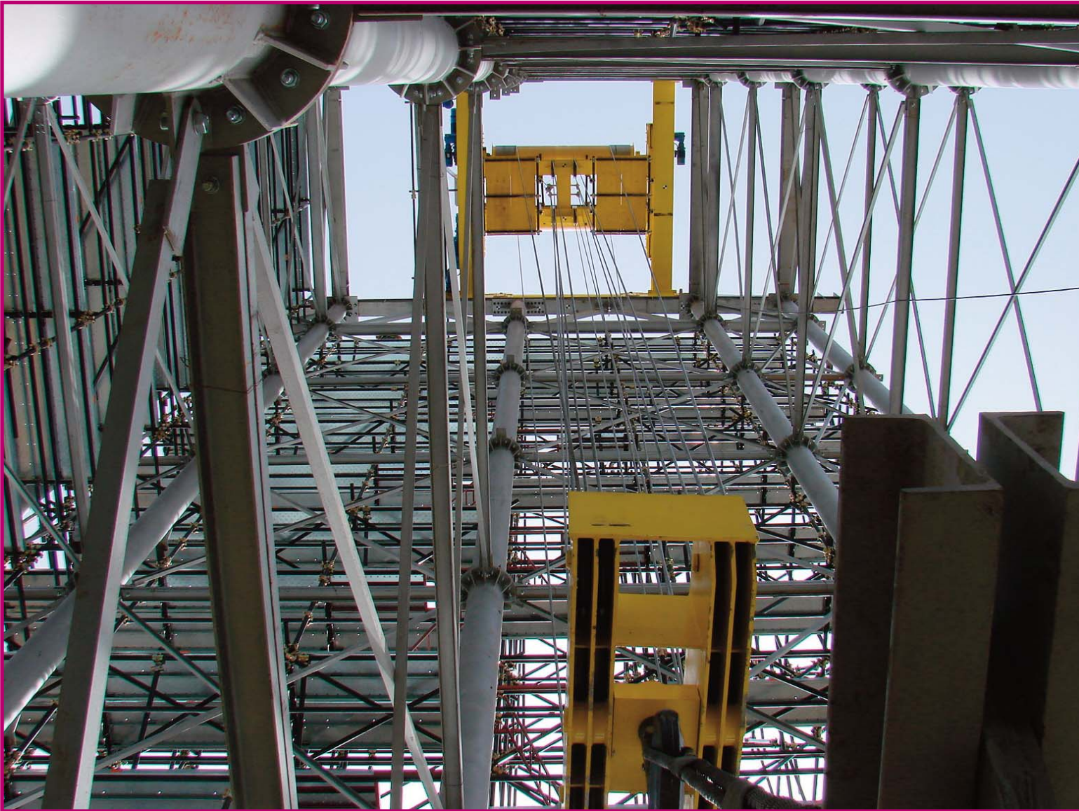
FIGURE 56 – VIEW FROM BELOW OF BRIDGE CRANE AND SUPPORTING STEEL CASTLE.
