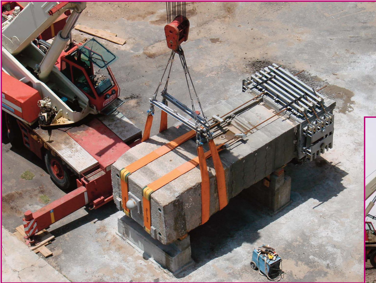
FIGURE 51 – THE BLOCK IS SECURED FIRMLY BEFORE HANDLING. FIGURE 52 – THE BLOCK IS LIFTED AND MOVED TO THE RAILS.
