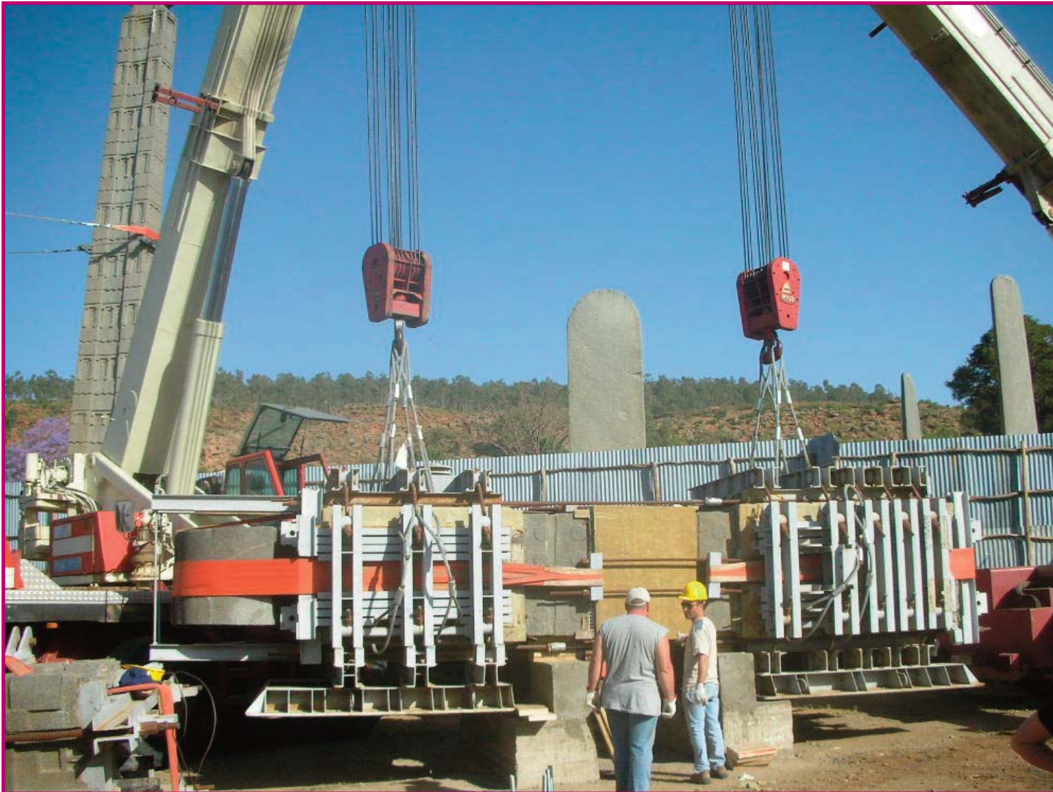
FIGURES 39 – HANDLING OF THE BLOCKS READY TO BE LIFTED UP
