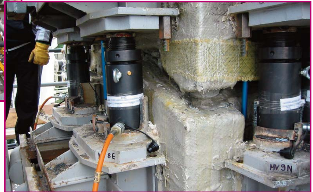
FIGURE 12 - DETAIL OF THE VERTICAL JACKS. THE JOINT BETWEEN TWO PORTIONS OF THE STELE, RIGHT AFTER ITS OPENING, IS ALSO VISIBLE.
