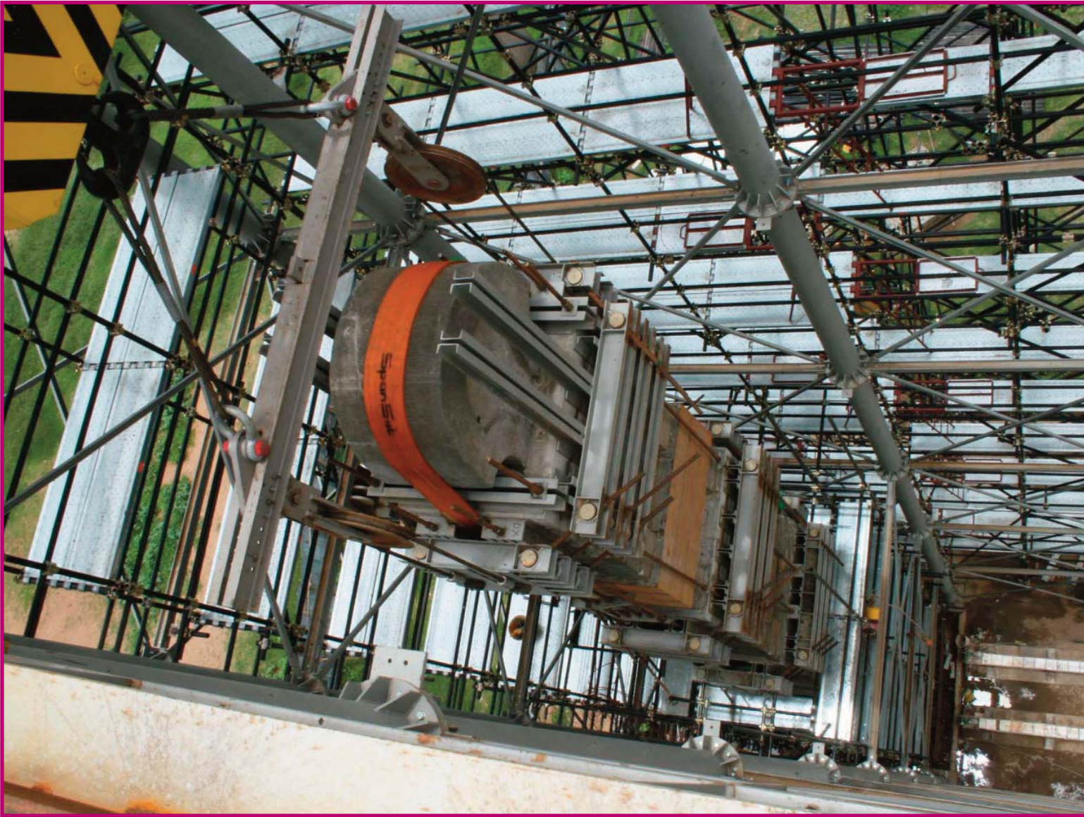
FIGURE 72 – LIFTING UP OF THE UPPER BLOCK (THIRD BLOCK). FIGURE 73 – THE FINAL CONFIGURATION OF THE STELE.
