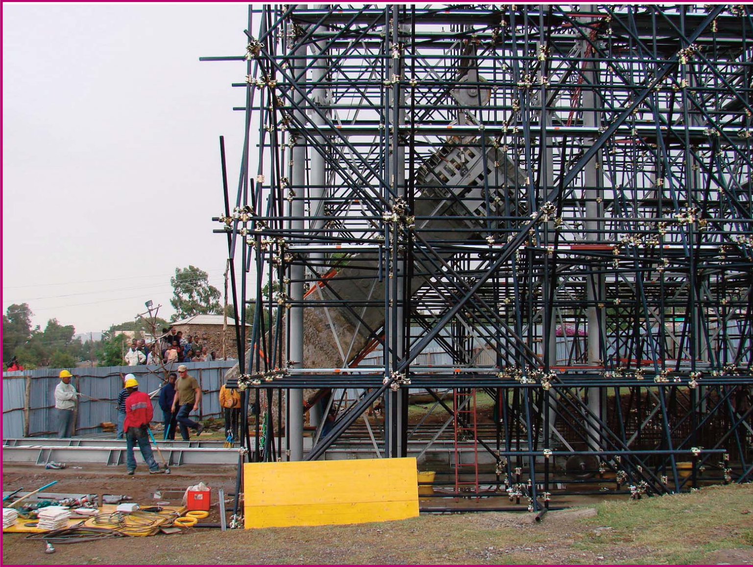
FIGURE 58 – THE LOWER PART OF THE BLOCK SLIDES ON THE RAILS WHILE THE UPPER PART IS LIFTED UP.
