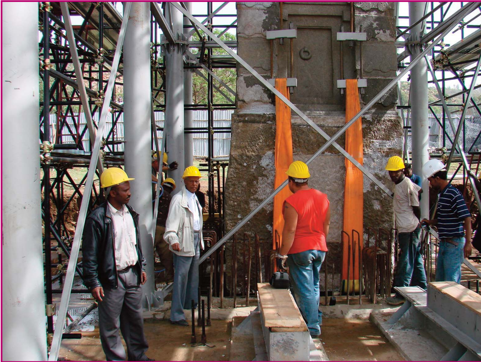
FIGURE 66 – FINAL POSITIONING OF THE BLOCK INTO THE HOUSING FOUNDATION.
