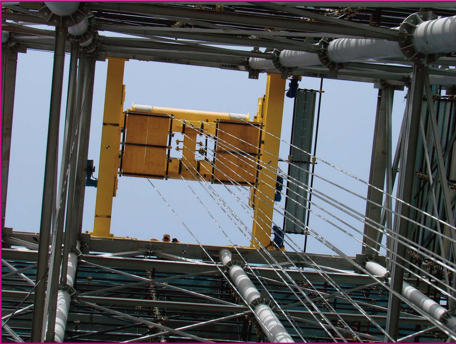
FIGURE 47 – THE BRIDGE CRANE FROM BELOW.
