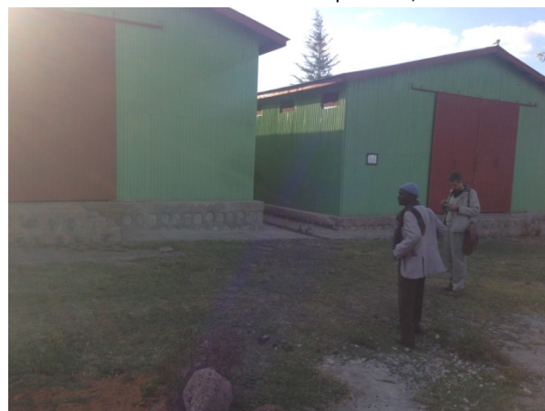
14. Dureti Tulu and Welta'e cooperatives warehouses
