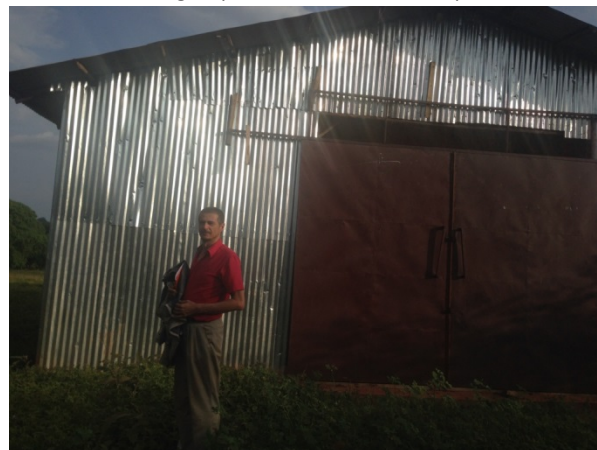
39. Irba cooperative warehouse
