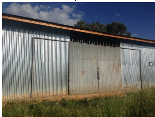
27. Oda Roba cooperative warehouse
