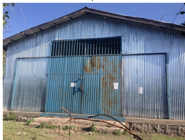
28. Ebisa cooperative warehouse
