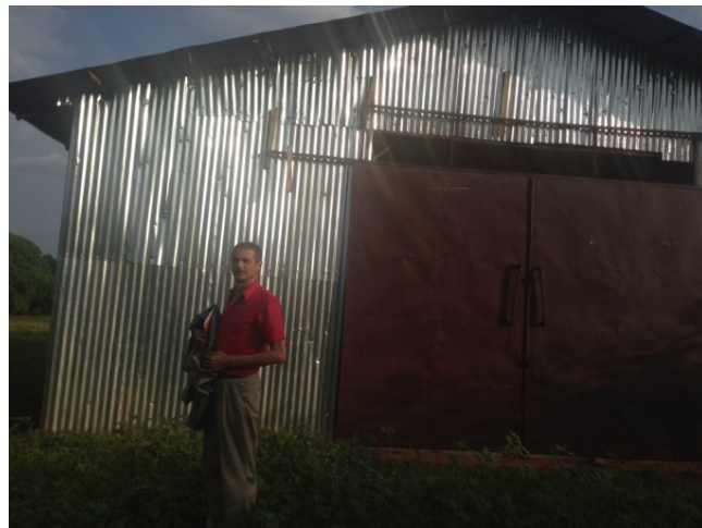
39. Irba cooperative warehouse
