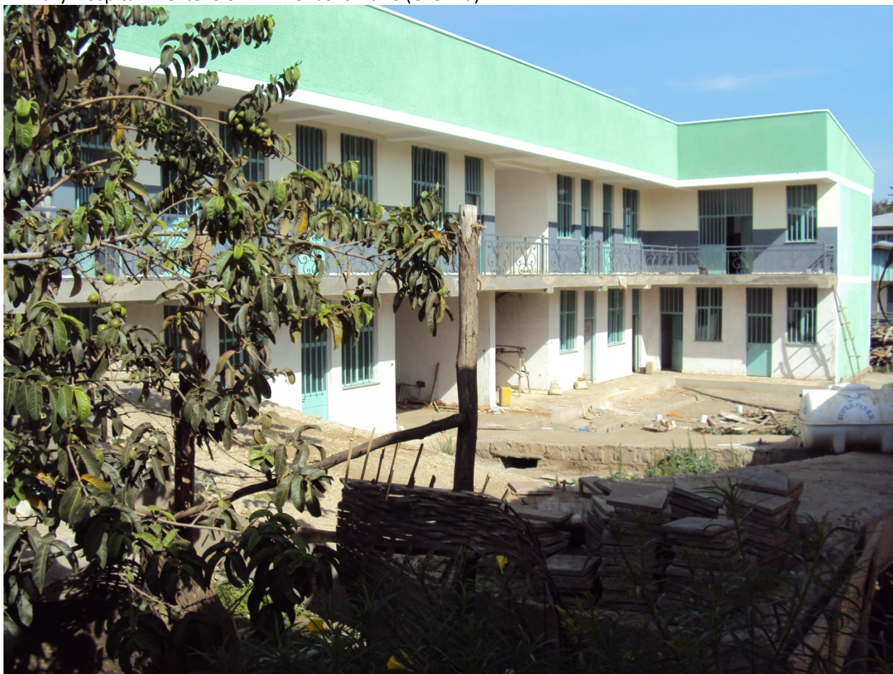
Primary Hospital in extension - PH Shashamane (Oromia)
