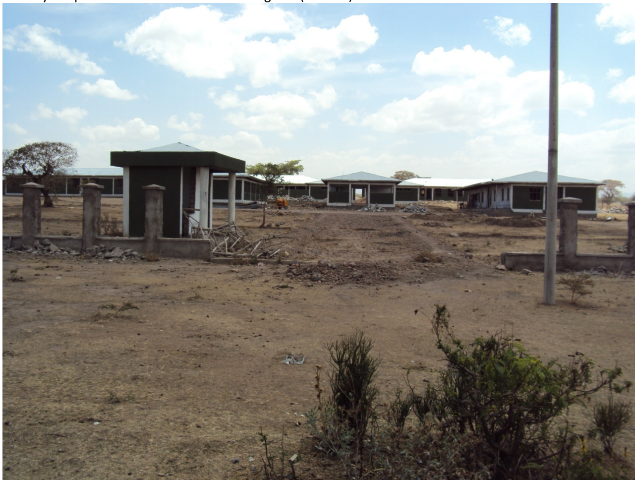
Primary Hospital under construction - PH Neghele (Oromia)
