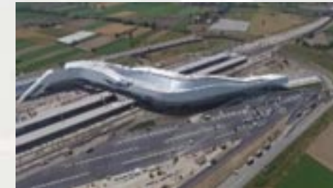
FS Naples HS Railway Station
