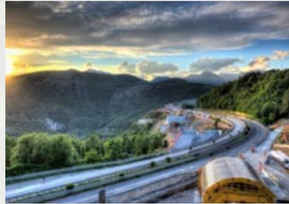
A3 Salerno – Reggio Calabria Highway - Italy
