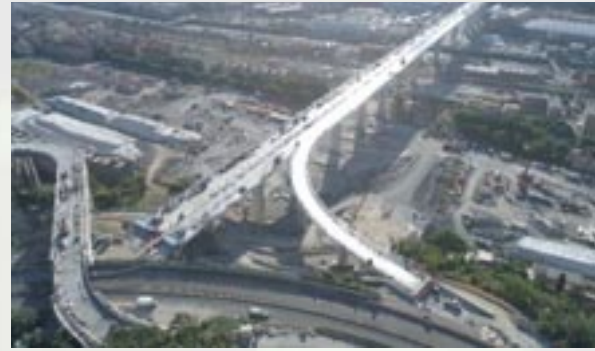
Genoa Saint George Bridge - Italy
