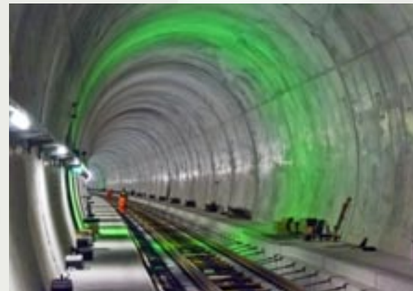
Monte Ceneri Base Tunnel - Switzerland
