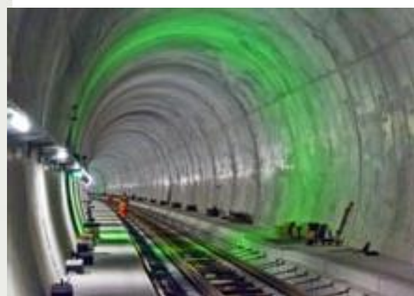
Monte Ceneri Base Tunnel - Switzerland
