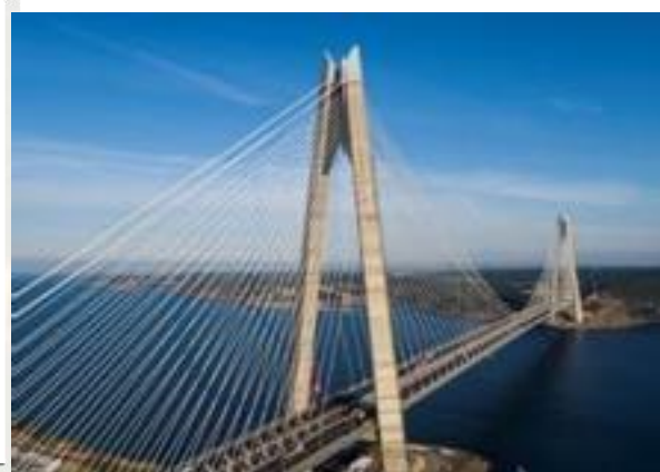
Third Bosphorus Bridge - Turkey
