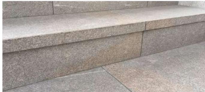
STONEWARE PAVEMENT - R11 not slip type - step with bullnose section
